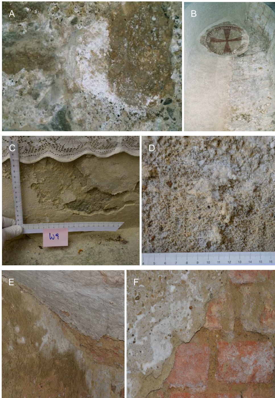
Figure 3. Salt efflorescences: A) detailed view on a salt formation and B) a salt-covered wall in the St. Virgil chapel (Vienna), C) detaching plaster material at the altar in the Saint Rupert chapel in Weißpriach (Austria), D) detailed view of salt efflorescences in the castle Rappottenstein (Austria), E) private garage with infiltrating water and salt formations, F) salt crusts in a private house (basement). All pictures were taken by Jörg Ettenauer.
