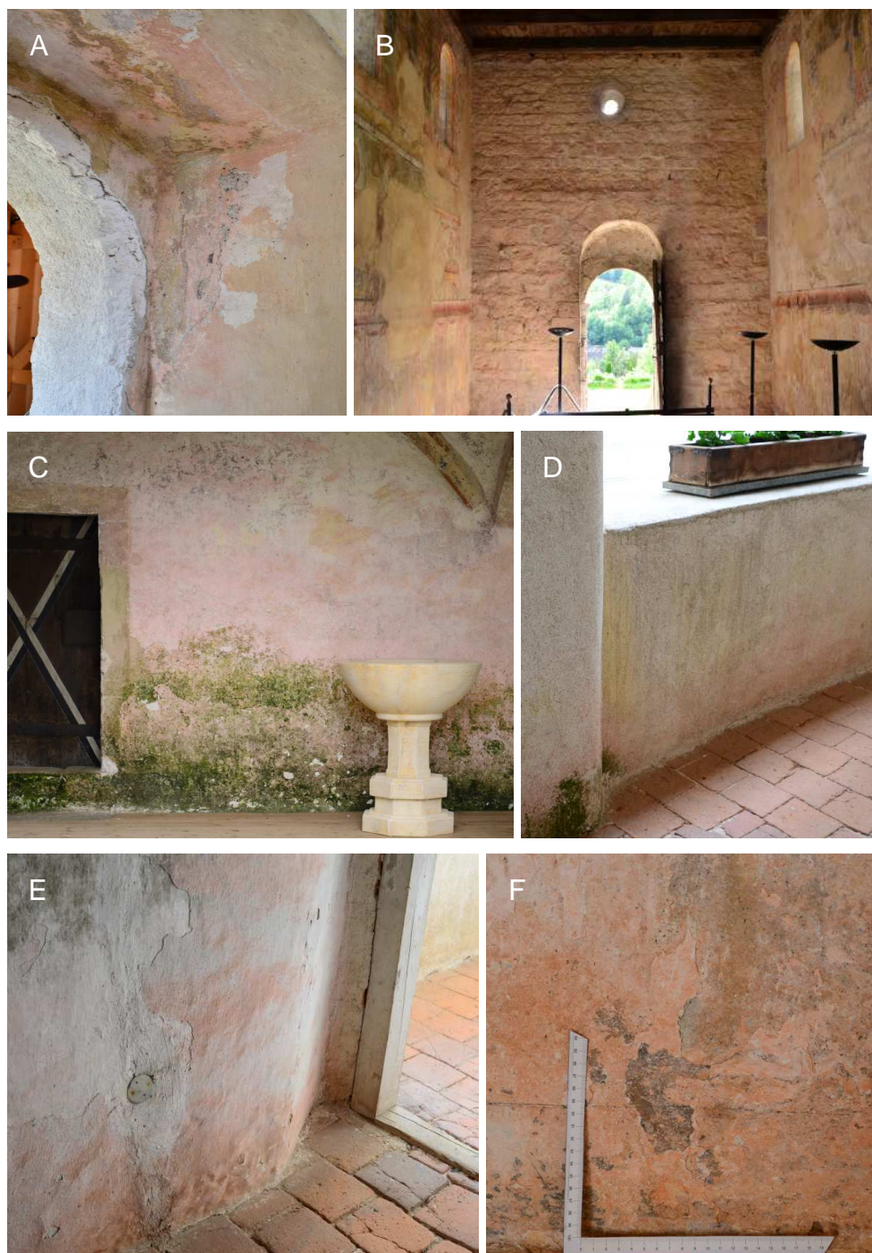
Figure 4. The rosy discolouration phenomenon: A) Entry arc and B) rosy stained inner west wall of the Johannes chapel in Pürgg (Austria), C) Inner courtyard and D) arcade of the castle Rappottenstein (Austria), E) doorway on the first floor of the castle, F) detailed view on rosy stained plaster material. All pictures were taken by Jörg Ettenauer.
