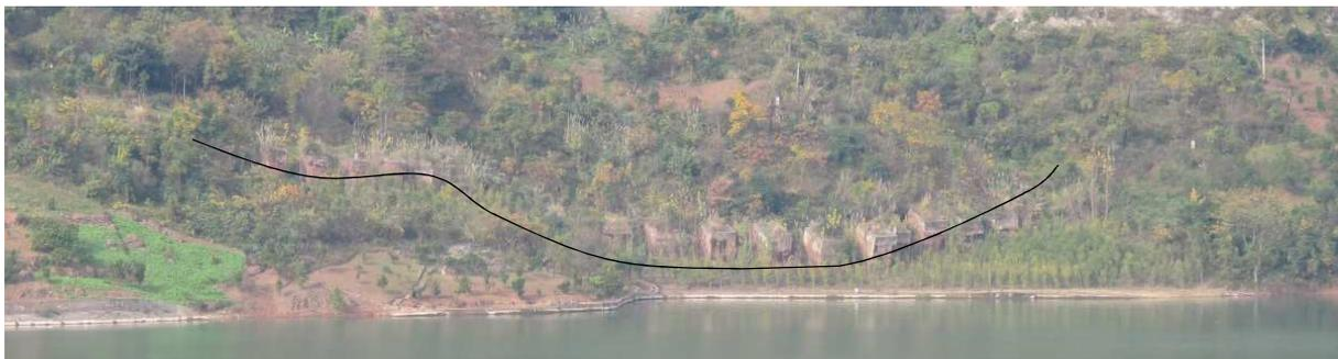
*Figure 23: Shi-jia-po landslide; black line: row of stabilising piles foundation (Photo: Mayrhofer 2012)*
