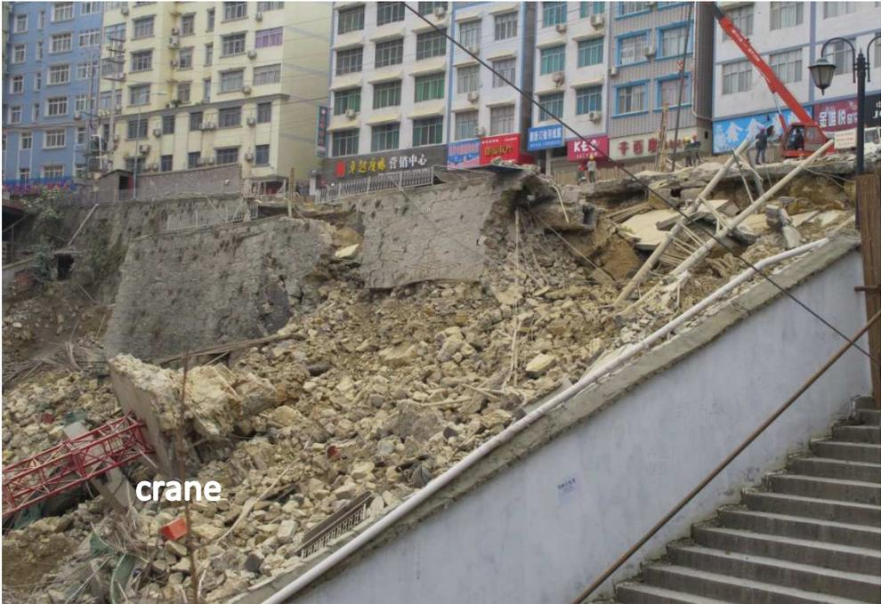
Figure 21: Slope failure in urban area of Badong (Photo: Mayrhofer 2012)
