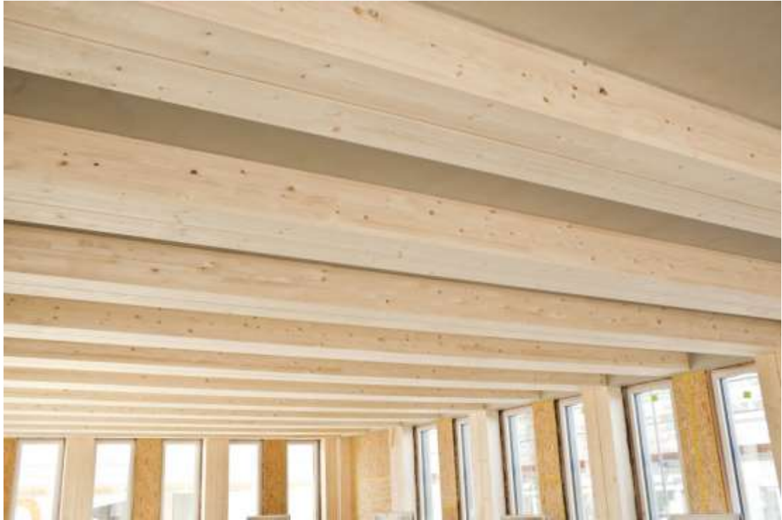
Figure 13: Visible load bearing timber components (source: Herman Kaufmann ZT GmbH 2012)
