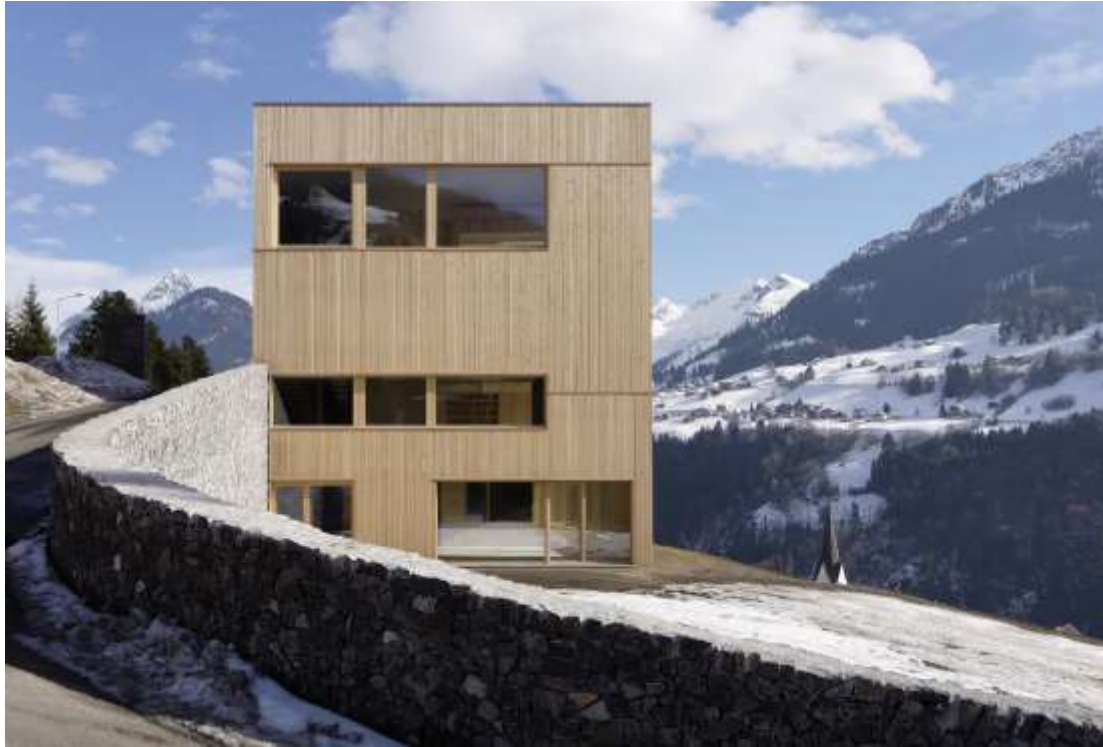
Figure 3: 4 storey perspective, south-west side, St.Gerold (picture: Hans Peter Schiess 2009, source Summer 2013)
