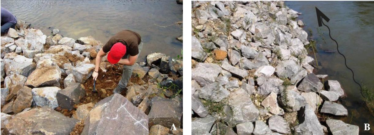
Figure 50: (A) Fielding the seedlings using a hand shovel. (B) Seedlings planted along the water line. Rio Pardinho, 04.2010. Picture, SUTILI.
