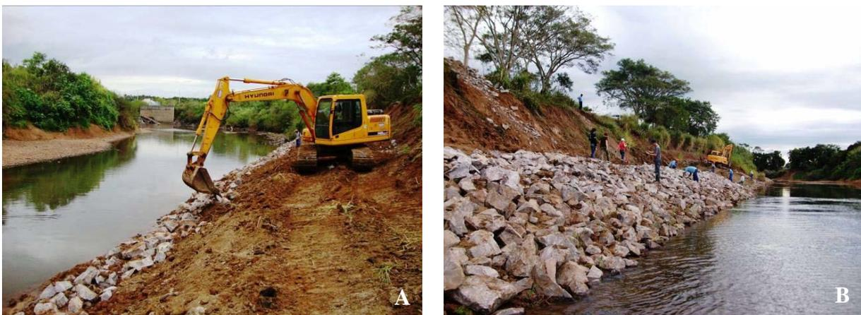
Figure 47: (A, B) Installation of riprap. Rio Pardinho, 04.2010. Picture, SUTILI.
