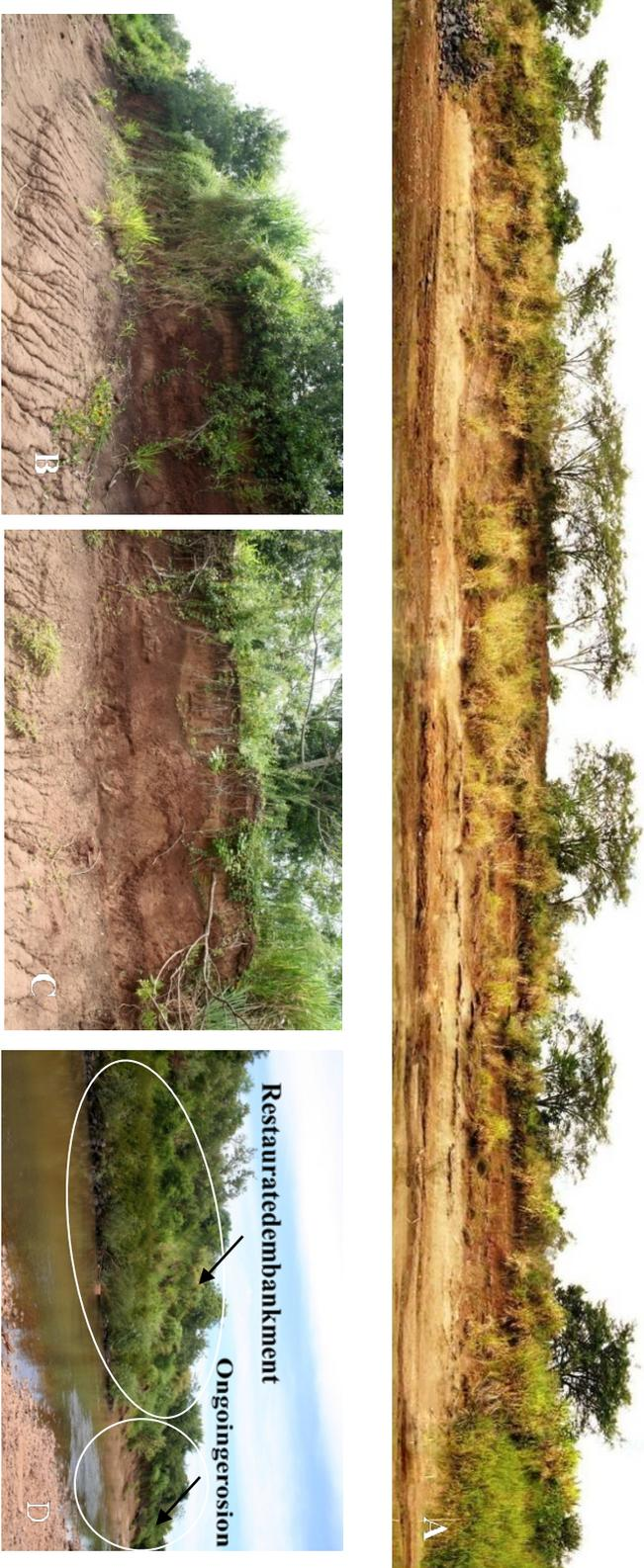
Figure 35: (A) Embankment before implementation of reinforcement works (SUTILI, 2010). (B, C) Erosive process, downstream of the intervention, observed in the year 2013. (D) Intervention and the eroding embankment downstream, in the year 2013, at the rio Pardino. Santa Cruz do Sul (A) 08.2010 (B,C,D) 01.2013.
