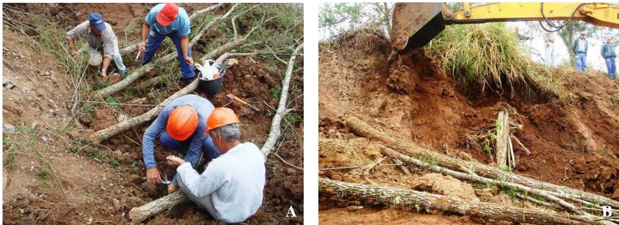
Figure 53: (A) Wooden poles (Eucalyptus). (B) The same stakes being buried 1.5 m deep and at an angle of 45° towards the slope. Rio Pardino, 05.2010. Picture, SUTILI.
