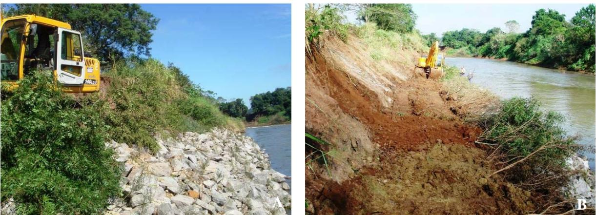
Figure 51: Installation of the hedge brush layer above the vegetated riprap. (B) After the shrubs are mounted, they are covered with a soil layer. Rio Pardinho, 04.2010. Picture, SUTILI.
