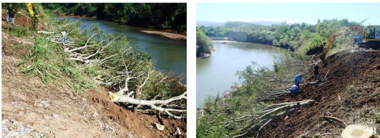
Figure 55: Anchored trees of *Enterolobium contortisiliquum*. (B) Shaping the slope angle. Rio Pardo, 05.2010. Picture, SUTILI.
