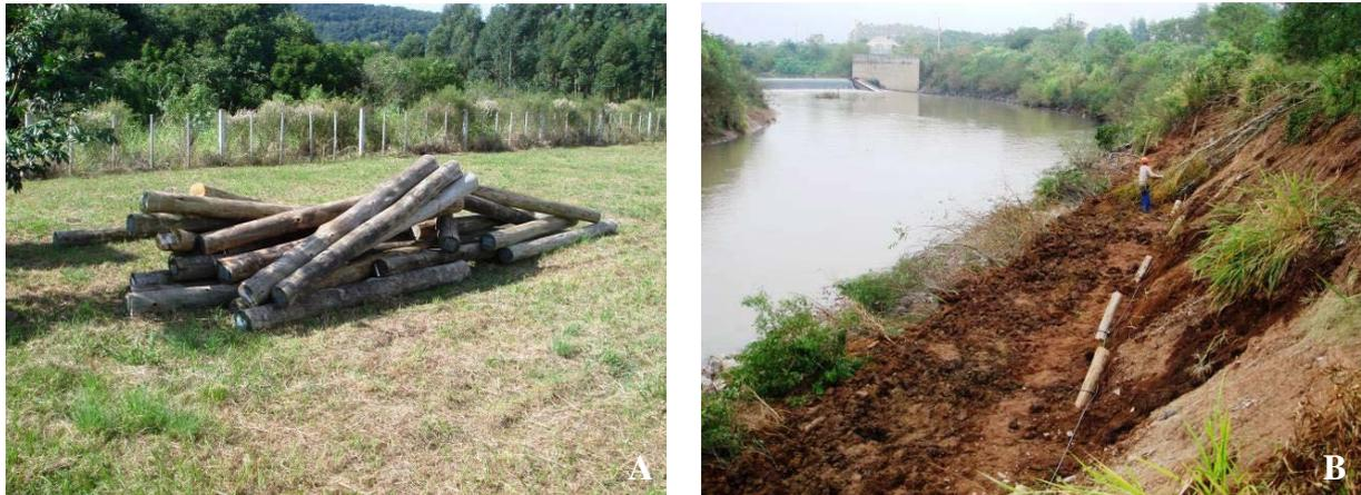
Figure 52: (A) Interconnecting willows with steel wire. (B) Mounting of a soil layer due to expectation of propagation. Rio Pardino, 05.2010. Picture, SUTILI.
