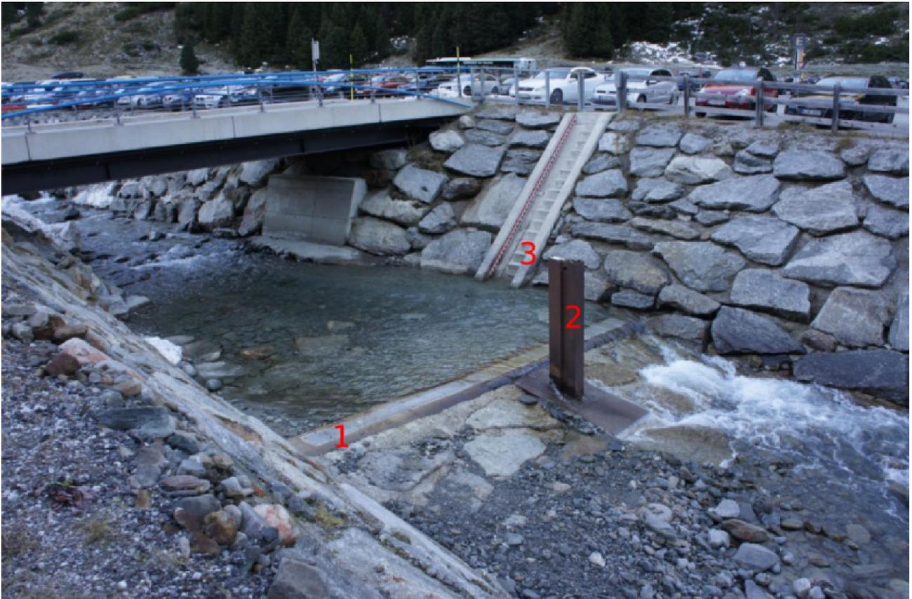
Fig. 3.4: geophone station in the Ruetz, 1: concrete sill with geophon plates in steel profile, 2: pillar for calibration basket, 3: stairs with visual water gauge (=location of pressure gauge)
