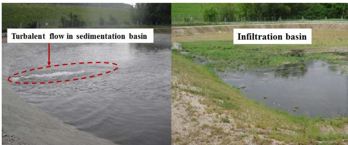
Figure 12. A photo depicting flow distribution for a runoff event on 10.06.2012 at GSA-A2; sedimentation (left) and filter basin (right).
