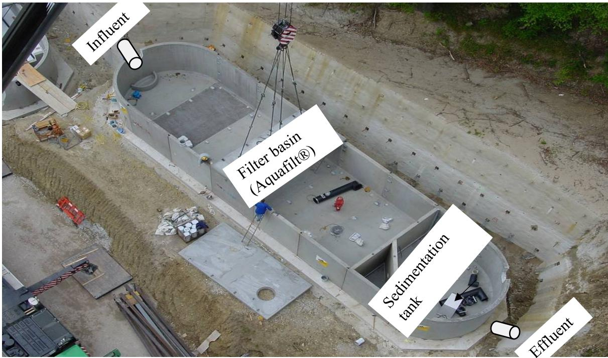
Figure 9. A picture of the filtration system for GSA-W catchment area.
