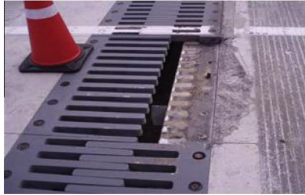
Abbildung 123 Failure of the finger-joint in Young-Bong bridge II, Korea in which the right plate popped up because of the failure of the anchor bolts, übernommen aus [20]
