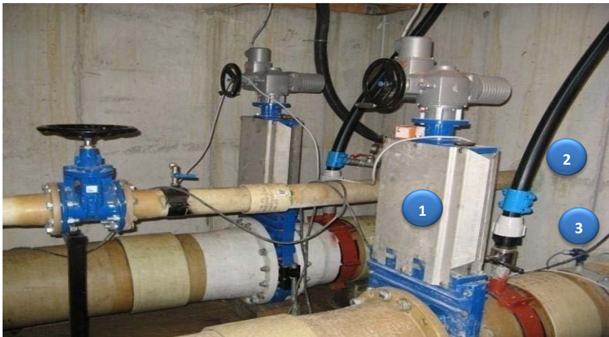
Figure 11. Technical overview- 1) knife gate valve; 2) water outtake for the three round basin, 3) temperature sensors (Auer, 2013)
