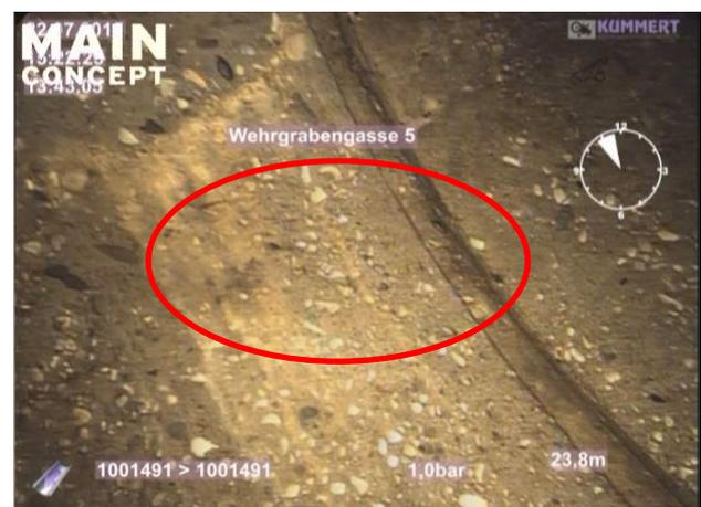
Abbildung 454: Beton DN500/800, TV-Kamera 3, Riss, 1mm
