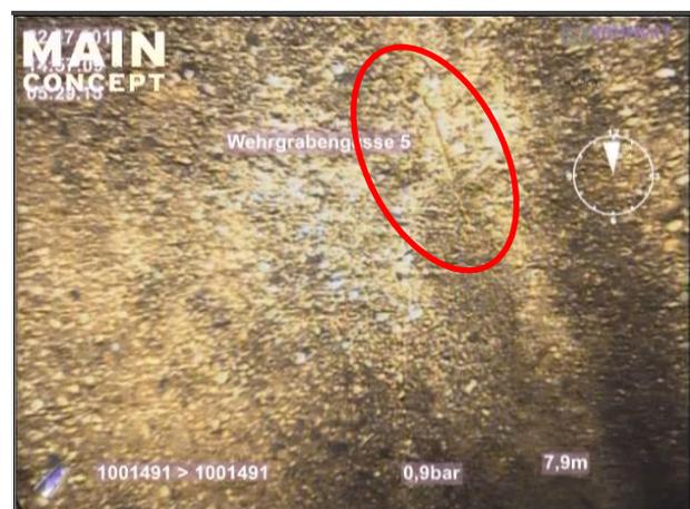
Abbildung 449: Beton DN500/800, TV-Kamera 3, Riss, 2mm
