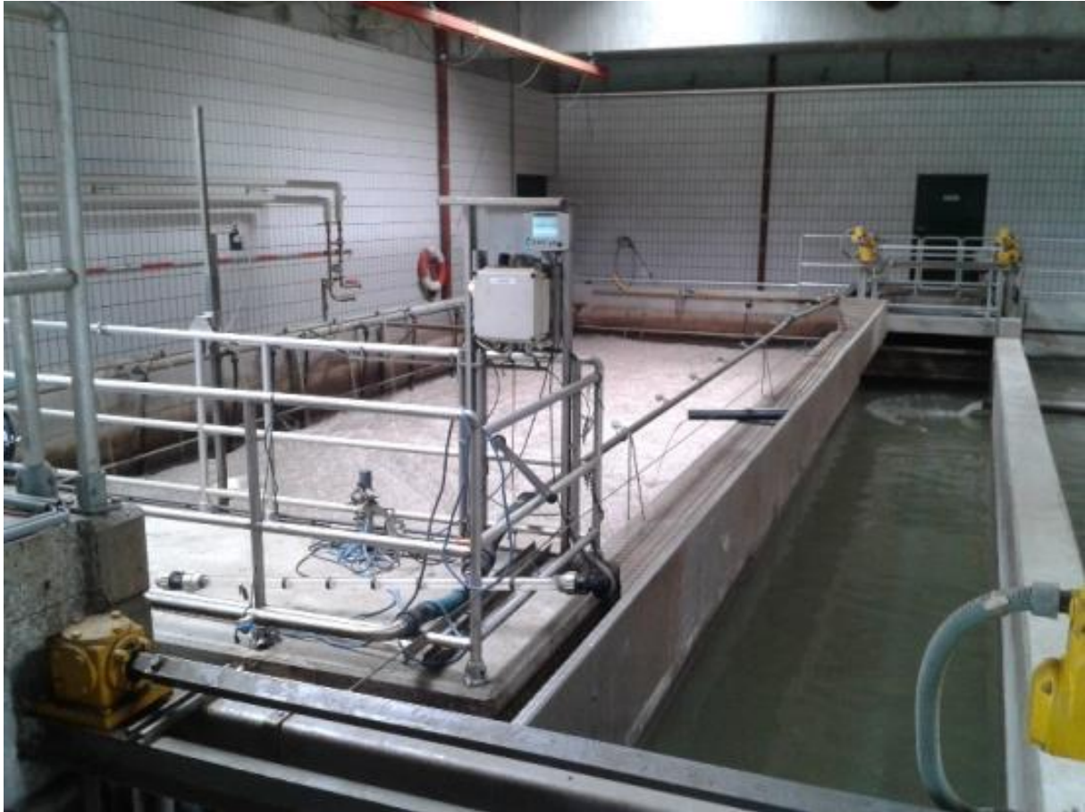
Figure 2: The source of inoculum, the DEMON® side stream treatment process at the WWTP Strass Tyrol (Weissenbacher et al. 2017)
