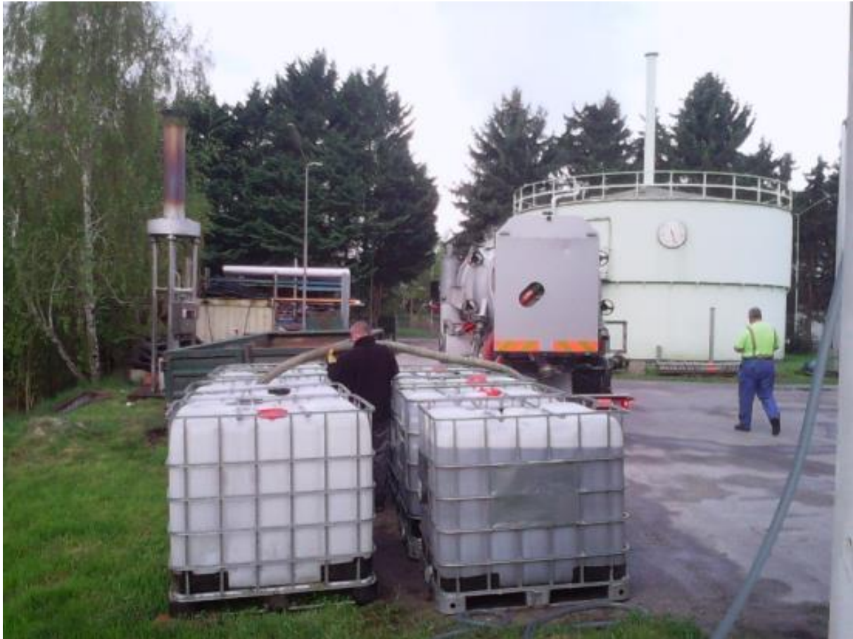
Figure 12: Loading of onsite storage of reject water collected in 10 m 3 IBC tanks (Weissenbacher et al. 2017).
