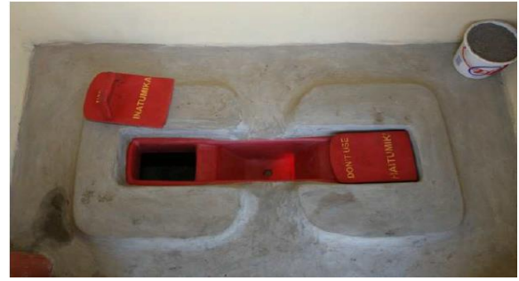
Figure 2 Picture of squatting pan from GIZ Kenya (2008) like it was installed in the EPP project and scheme of UDDT after Rieck et al., 2012.
