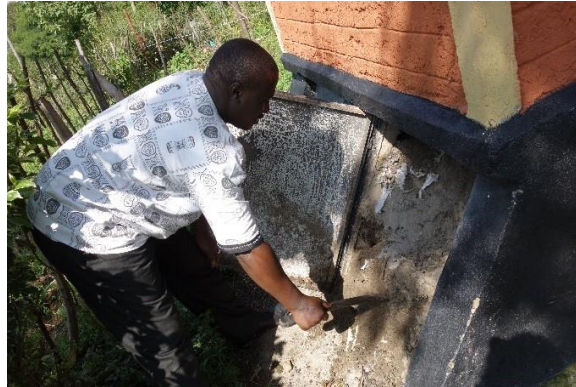
Figure 7 Picture of dried faecal matter in faeces chamber, taken during the questionnaire survey.
