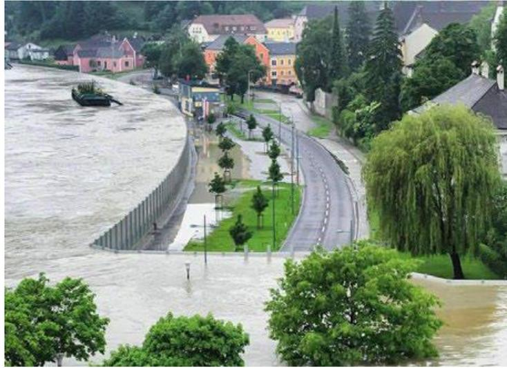
Figure 6: Mobile protection walls along the river Danube in Krems, Lower Austria (from Habersack et al. 2015, p. 45).
