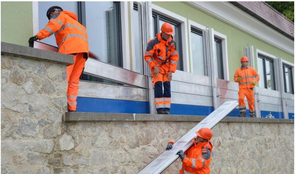
Figure 5: Construction of mobile water barriers for a house along the river Danube in Schärding, Upper Austria (from Habersack et al. 2015, p. 45).
