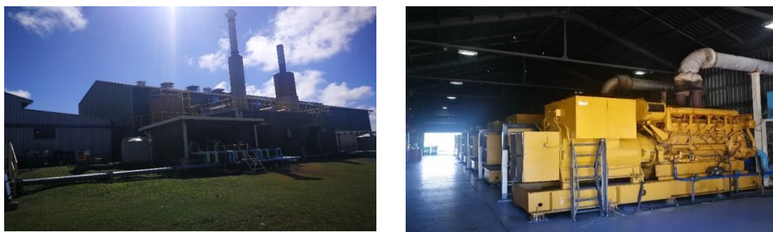
Figure 5.4: TPL's Popua Power Station and Caterpillar (CAT-1750kVA-50Hz-CP_C) Generator, own representation
