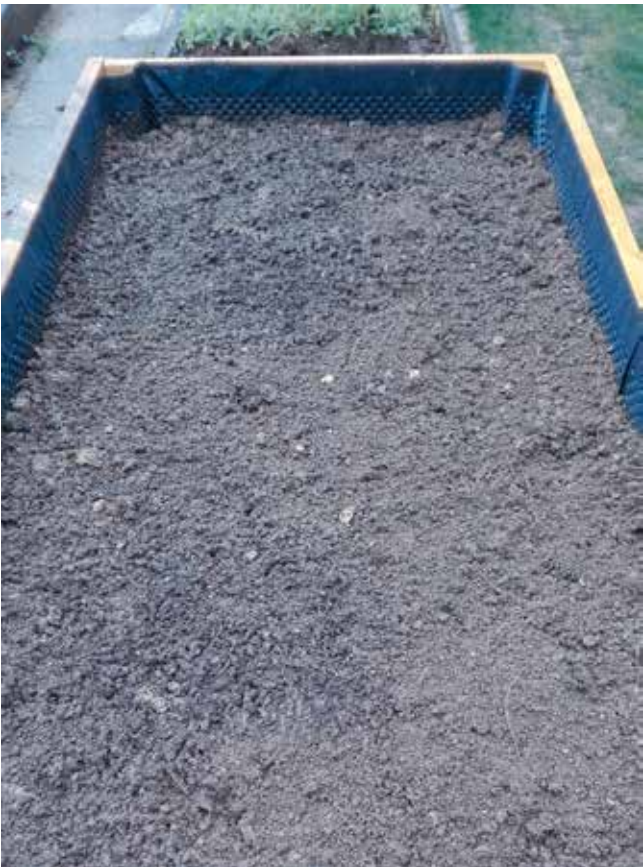
Figure 24. Stormwater planter with clay based substrate (Edward Gunn).
