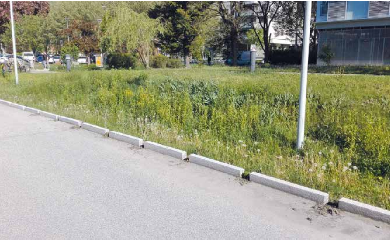
Figure 12. Rain garden collecting surface run off from a road, at the University of Innsbruck (Edward Gunn).
