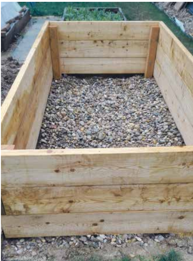
Figure 22. Wooden construction of the stormwater planter for the trial (Edward Gunn).
