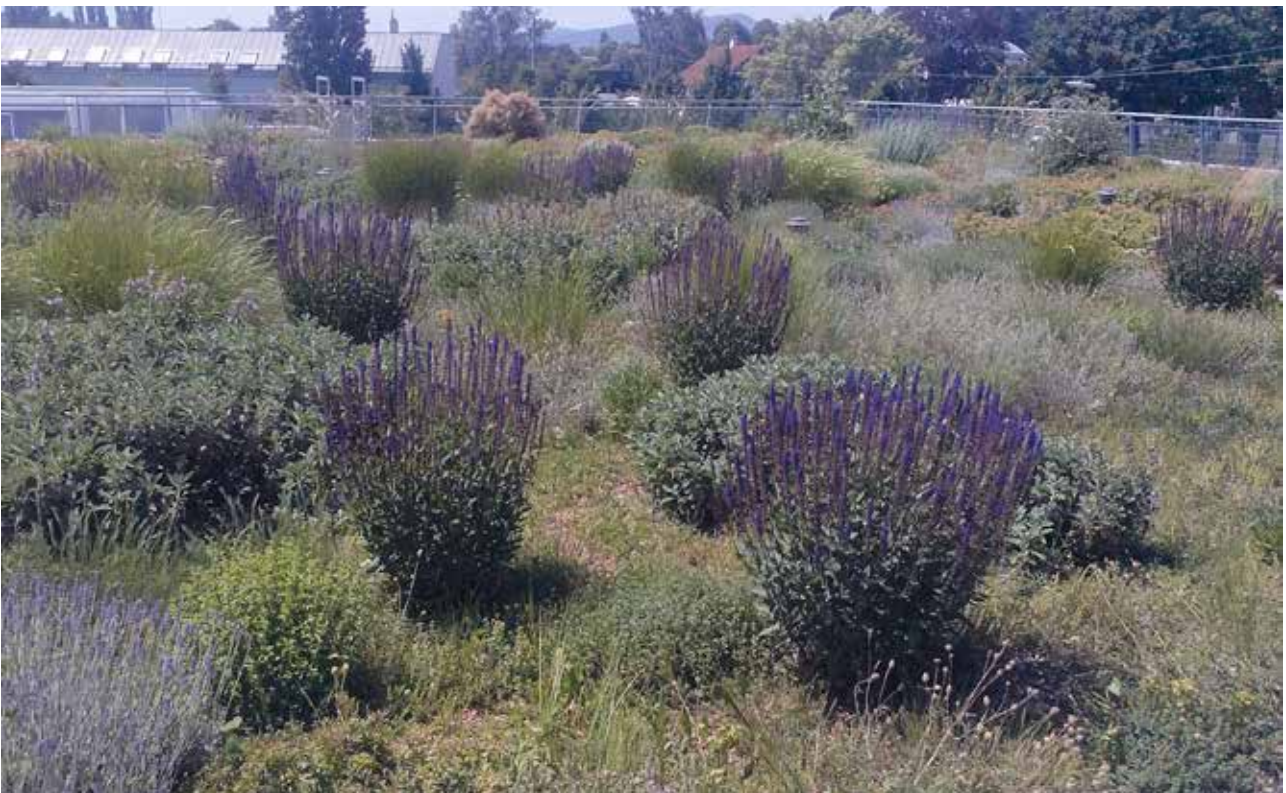
Figure 2. Intensive (green) roof with a 25 cm substrate layer on top of a 5 cm drainage layer, the planting includes perennials, grasses and small shrubs; Horticultural School (HBLFA Gartenbau Schönbrunn) Vienna (Edward Gunn).
