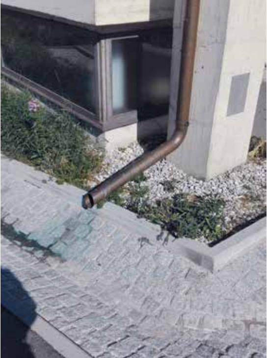
Figure 15. Gully (which then flows into a swale) collecting rainwater from a roof downpipe, at the University of Innsbruck (Edward Gunn).
