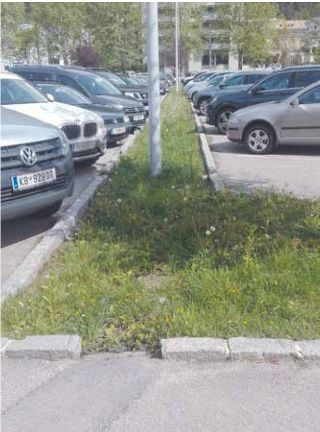
Figure 13. Swale collecting rainwater from a car park, at the University of Innsbruck (Edward Gunn).
