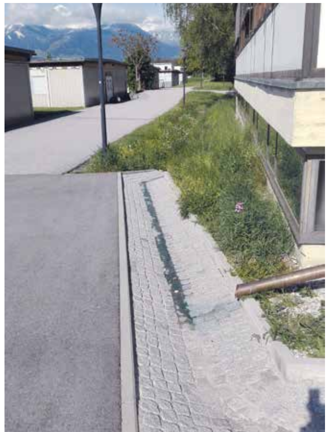
Figure 8. Stage 2 of a stormwater chain: gully then flows into a swale, at the University of Innsbruck (Edward Gunn).
