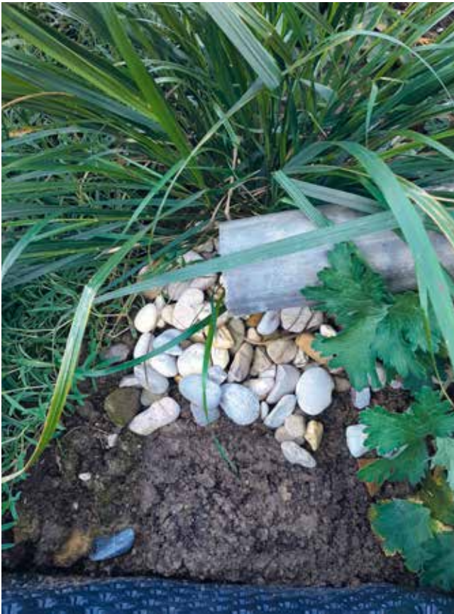
Figure 28. Pebbles placed by water inlet to prevent erosion (Edward Gunn).
