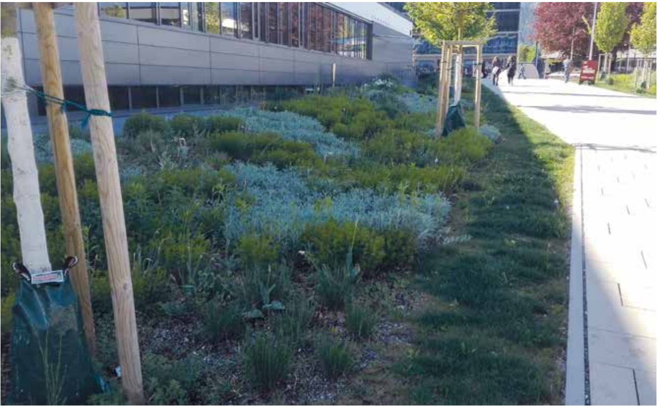
Figure 14. Raingarden collecting rainwater from a pedestrian area, at the University of Innsbruck (Edward Gunn).
