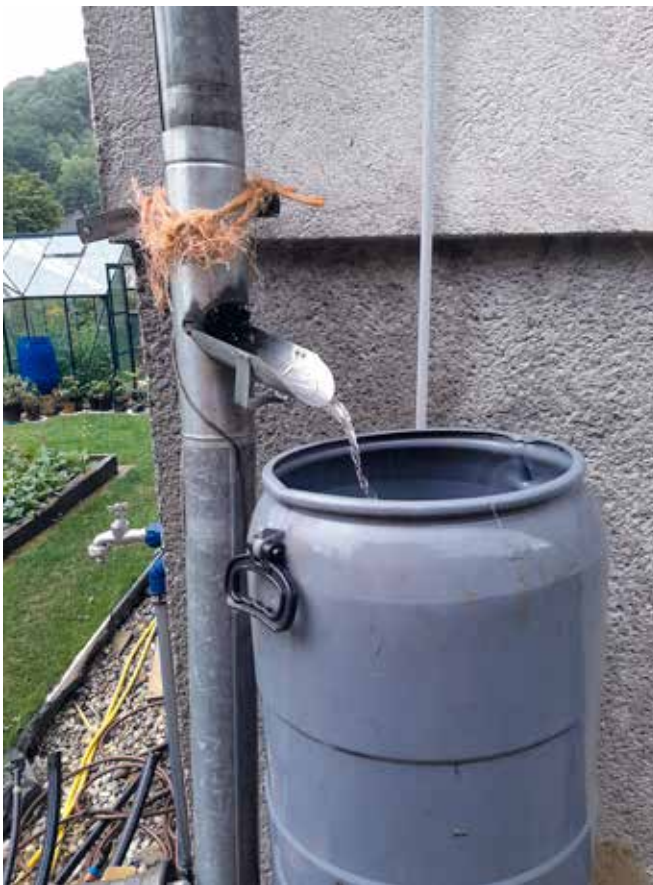
Figure 6. Water barrel collecting rain water from a house downpipe (Edward Gunn).
