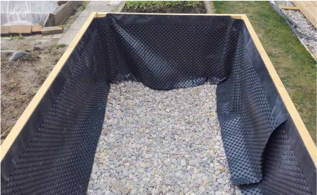
Figure 23. Studded plastic added to stormwater planters (Edward Gunn).
