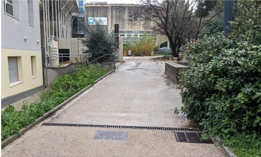
Figure 4: Outfall of the observation catchment through a rain channel covered by a trench drain grate and draining into a catchpit.
