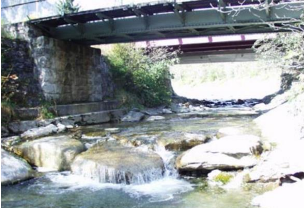
Figure 28: Example of a not fishpassable transverse element downstream a bridge (source: Office of the Salzburg Provincial Government, Water Protection Department)
