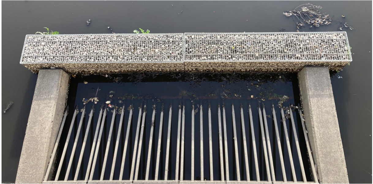
Figure 3: Rectangular stone structure installed to break the velocity and trap bigger sediments
