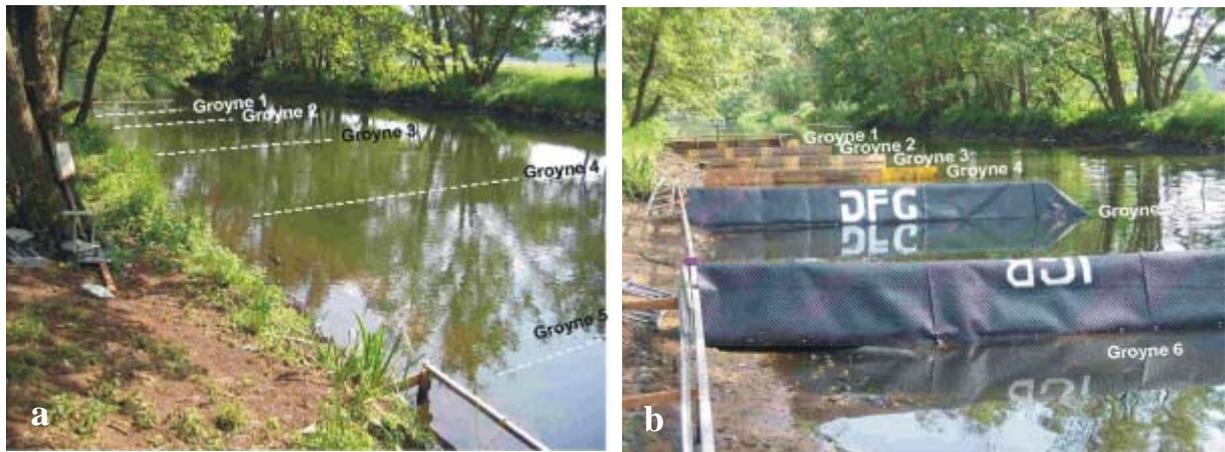
**Figure 3.8:** River reach (river Spree) with installed groynes: submerged (a) and emerged conditions (b), 2007.
