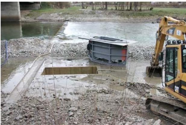
**Figure 21:** The hydraulic lift trap before installation
