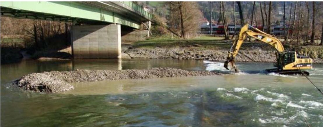
**Figure 65:** Maintenance operation at fixed slot samplers (April 2010)
