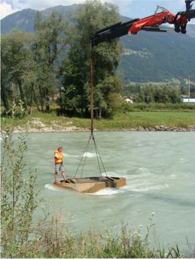
**Figure 64:** Maintenance operation at hydraulic lift trap (August 2009)
