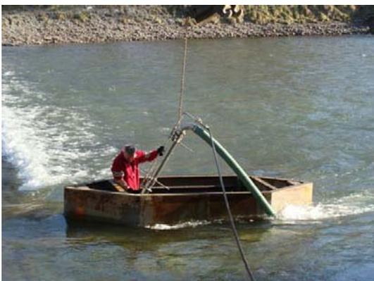
**Figure 39:** Removal of sediment accumulations using an airlift pump
