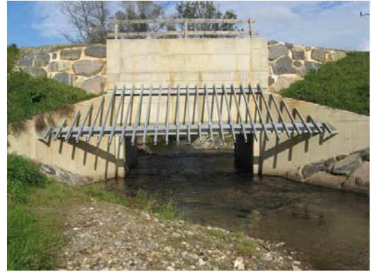
Figure 11: ecological orientated bottom outlet, left: structured bed of a culvert, right: (short culvert with a large cross-sectional area)
