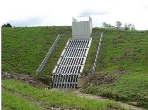
Figure 8: location of the control section - in the middle of the bottom outlet
