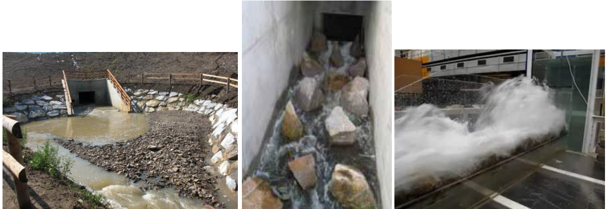
Figure 12: left: absorption basin - bed load sedimentation, middle and right: energy dissipation along a rough bed in the culvert
