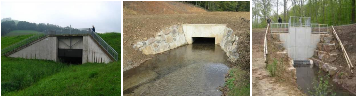
Figure 4: material of intake structures left: concrete, middle: block reinforcement, right: gabioni
