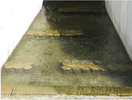
Figure 11: ecological orientated bottom outlet, left: structured bed of a culvert, right: (short culvert with a large cross-sectional area)
