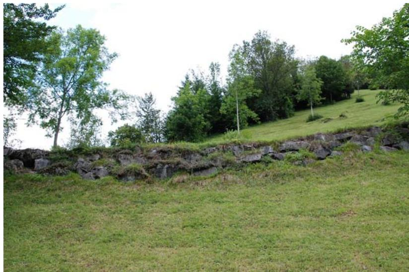
Abb. 20: Blockwurf 40B100 (© Gehring/Locher)
