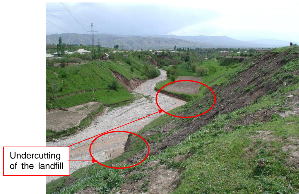
Figure 3.6: Old Dushanbe Landfill: Slope (height 25 m) at the river side (looking downstream)
