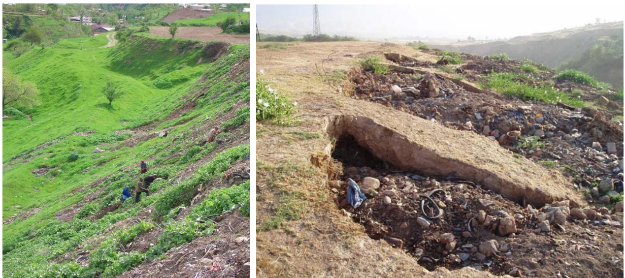
Figure 5.28: Undercutting of slope and excavation by people and exposure of waste possibly through excavation and erosion at the top of the riverside slope
