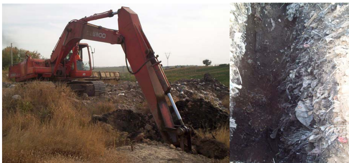
Figure 5.9: Pit excavation on the Ahangaranskaya Landfill
