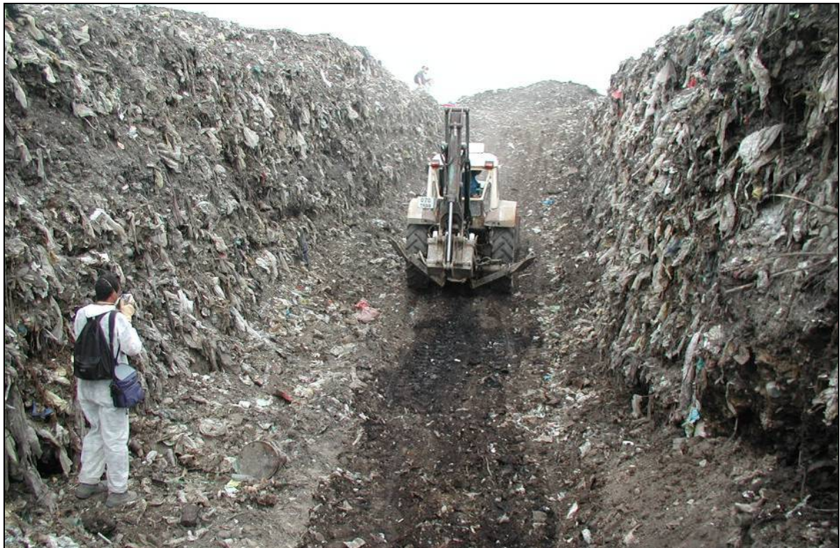
Figure 5.35: Trench in the old part of the landfill, depth approx. 6 meters
