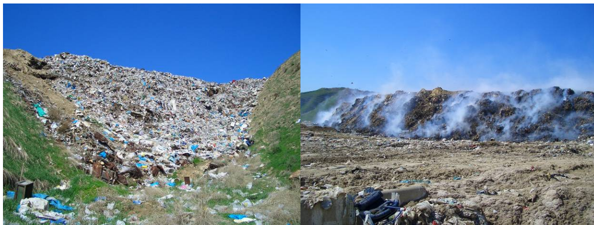
Figure 5.7: Loosely dumped waste should be placed in layers with proper compaction and side/top cover.
