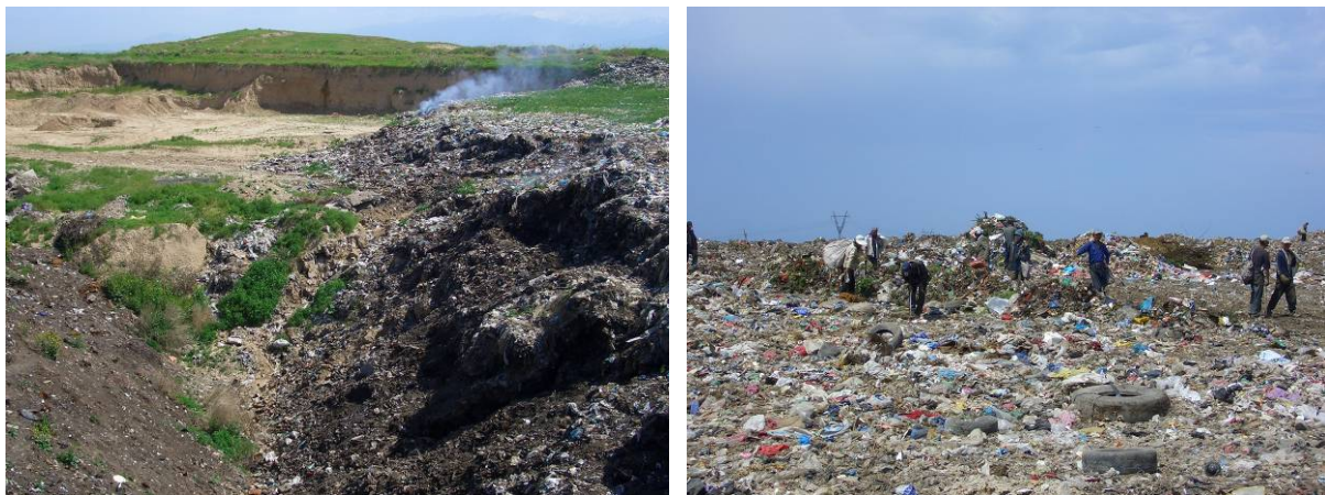
Figure 5.15: Slopes of the landfill should be flattened and compacted. Areas currently not used for disposal should be covered temporarily.
