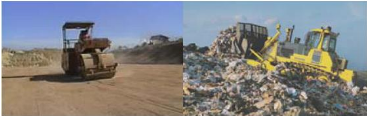
Figure 4.13: Engineered landfill (preparation of base sealing and waste compaction)
